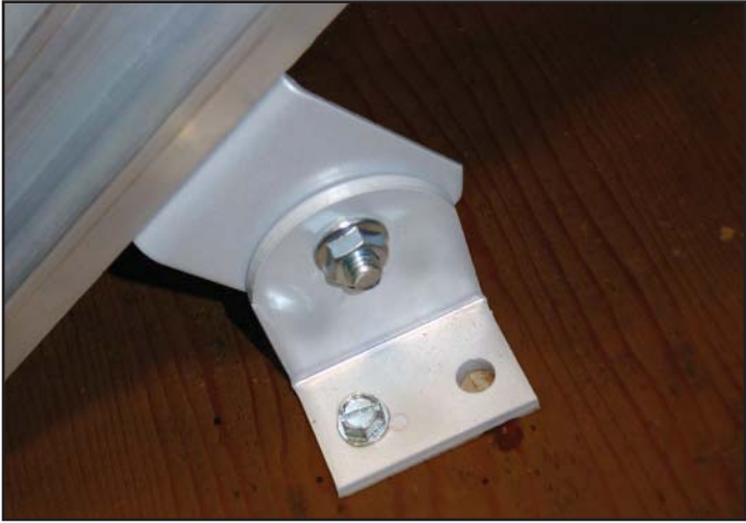
Track Bracket installed.
