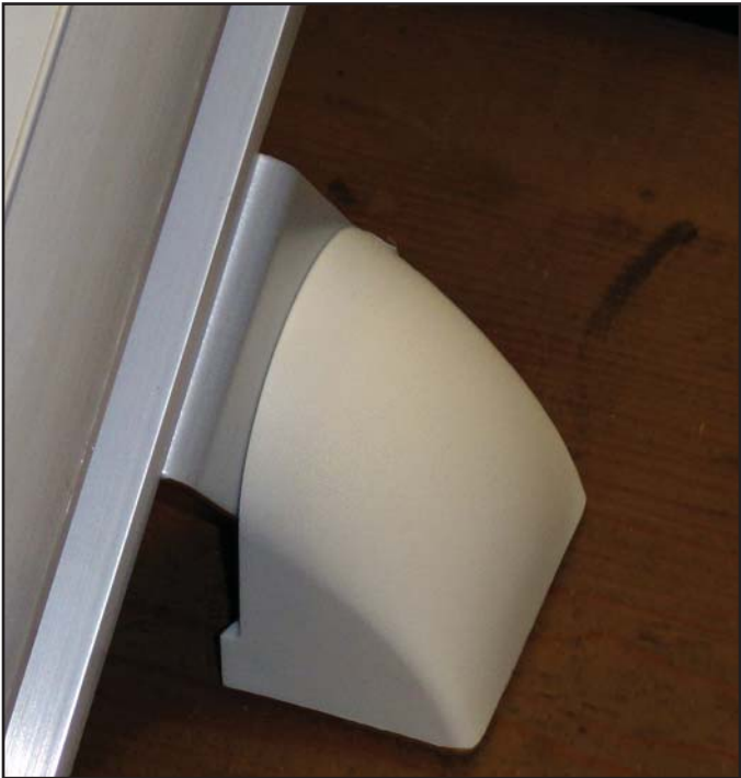
Track Bracket cover installed.
