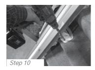
**STEP 10:** Fasten down the near corner of the lower bracket using a drill that has extensions at least ten-inches long and a 3/8" socket.
